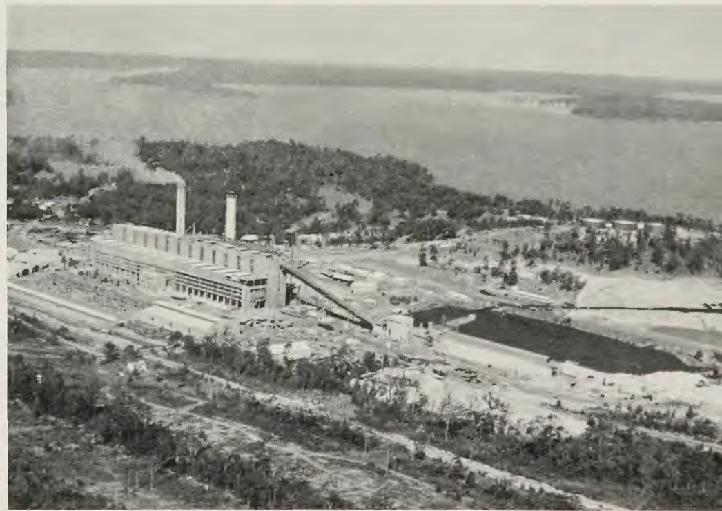
Electricity power station at Wangi, with Lake Macquarie in the background.
