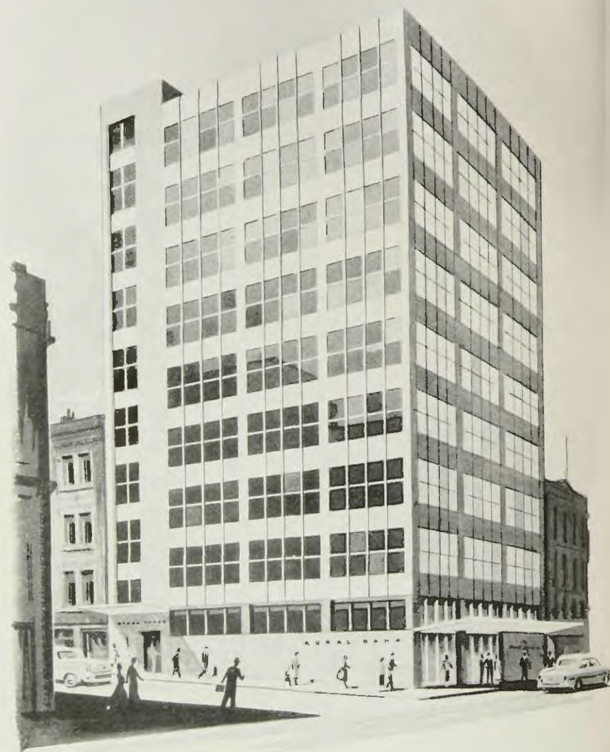
The new Rural Bank building, on the corner of Hunter and Bolton Streets Newcastle.
