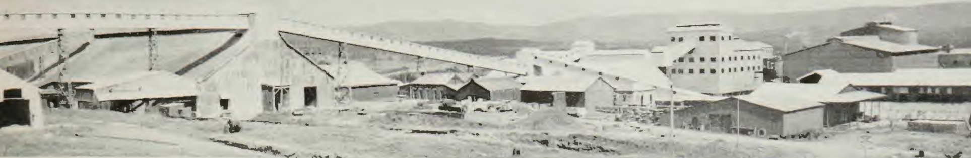
General view of the Sulphide Corporation's works at Cockle Creek.
