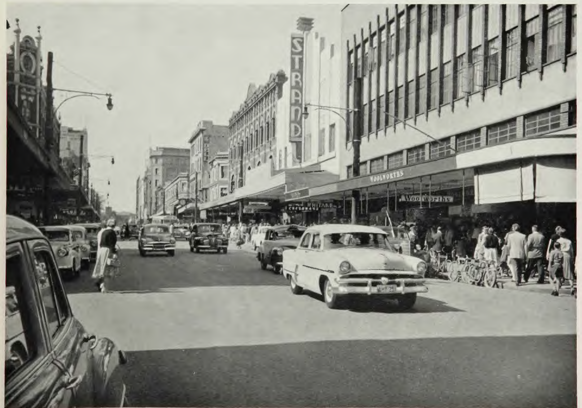
Hunter Street, looking east, with City Council properties in the foreground.
