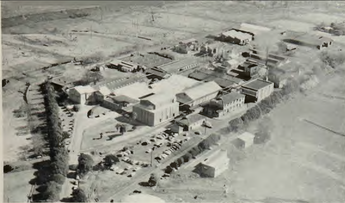
Aerial view of Abattoir buildings and portion of property.
