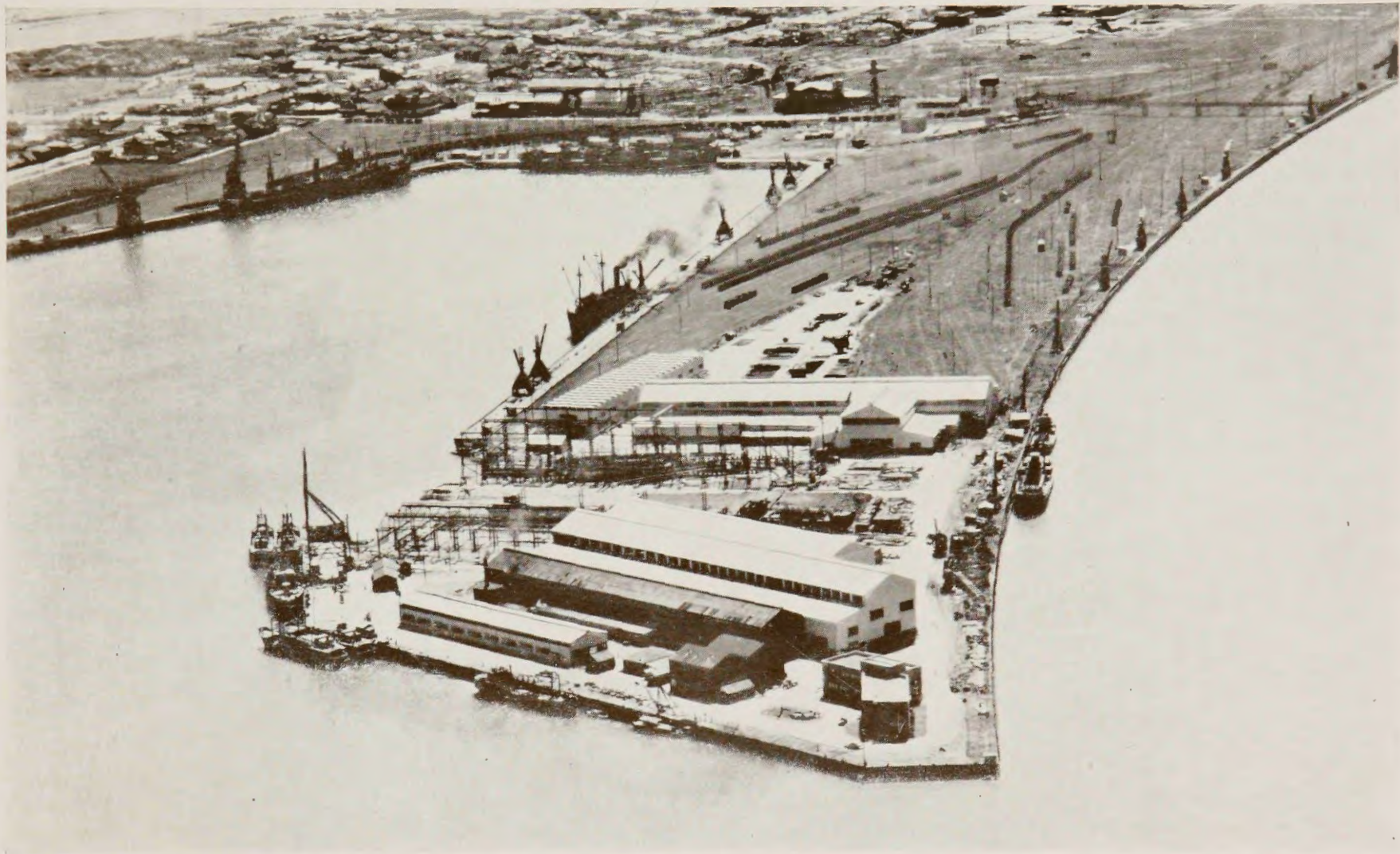
AERIAL VIEW OF DOCKYARD — MARCH, 1944 Looking North-West.
