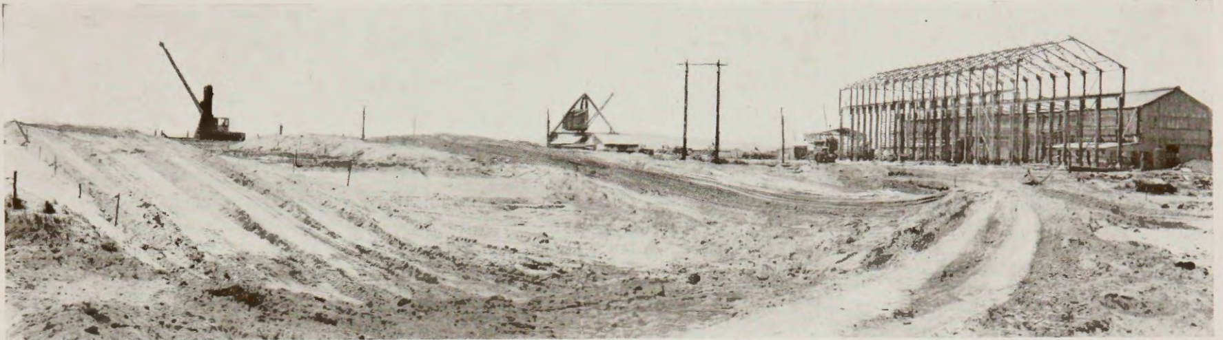
COMMENCEMENT OF CONSTRUCTION. [March, 1942.] Grading of Building Berths in foreground—Heavy Machine Shop Structure on right.
