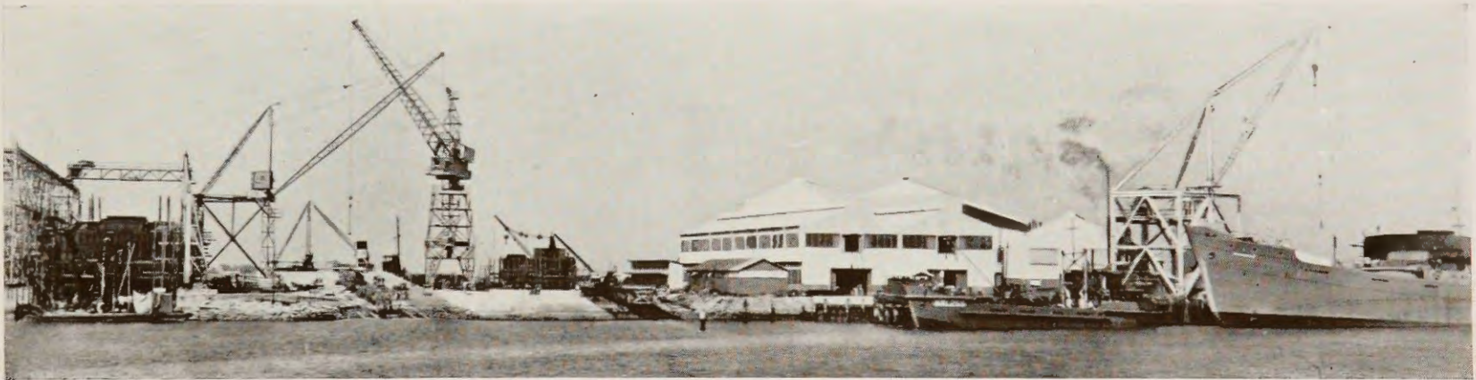
VIEW SHOWING Nos. 2, 3 and 4 BUILDING BERTHS AND VESSELS AT FITTING-OUT WHARF.
