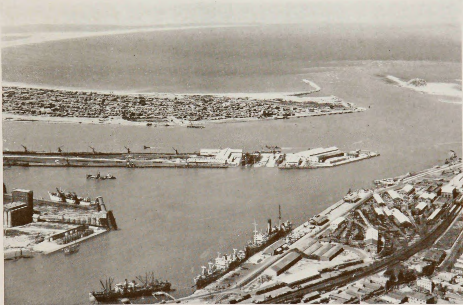
GENERAL VIEW OF DOCKYARD LOOKING NORTH-EAST. Showing entrance to Harbour.
