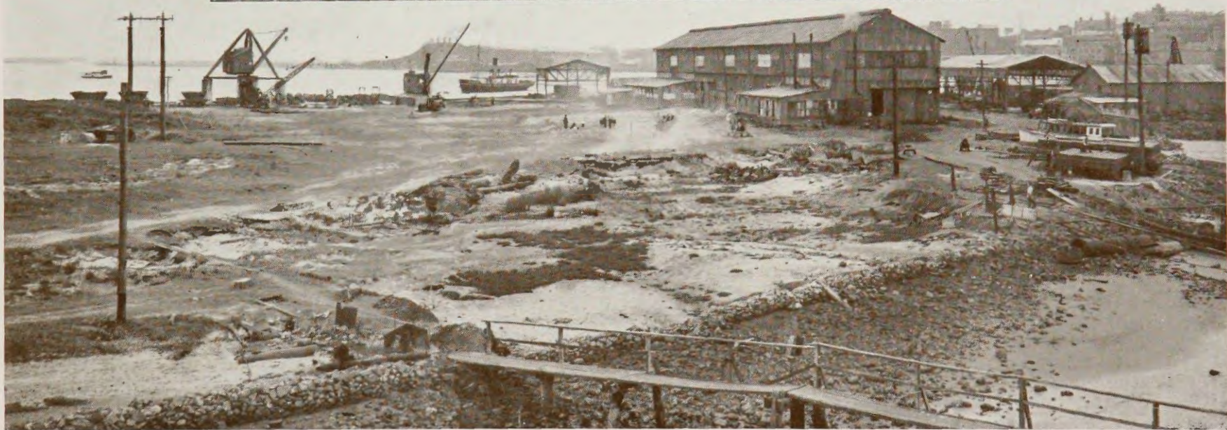
VIEWS OF SITE PRIOR TO COMMENCEMENT OF CONSTRUCTION. [January, 1942.]
