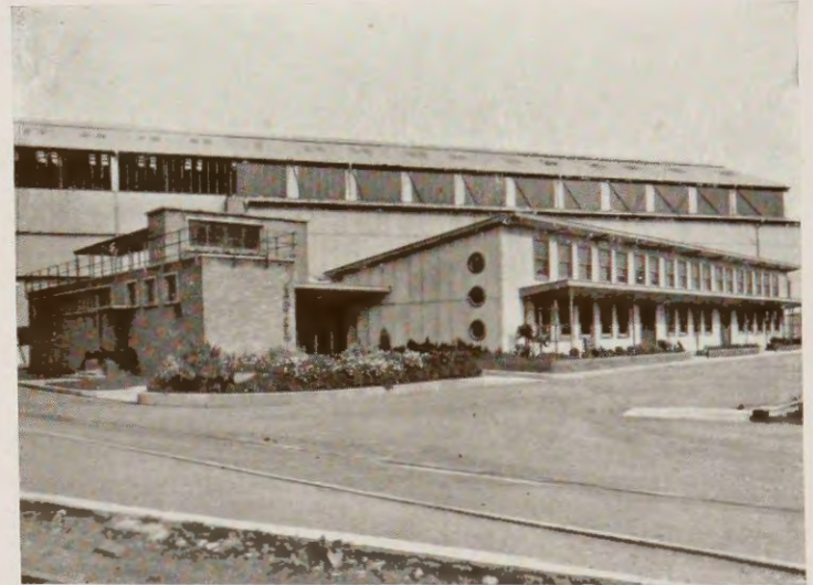
WORKMEN'S ACCOMMODATION BUILDING.
