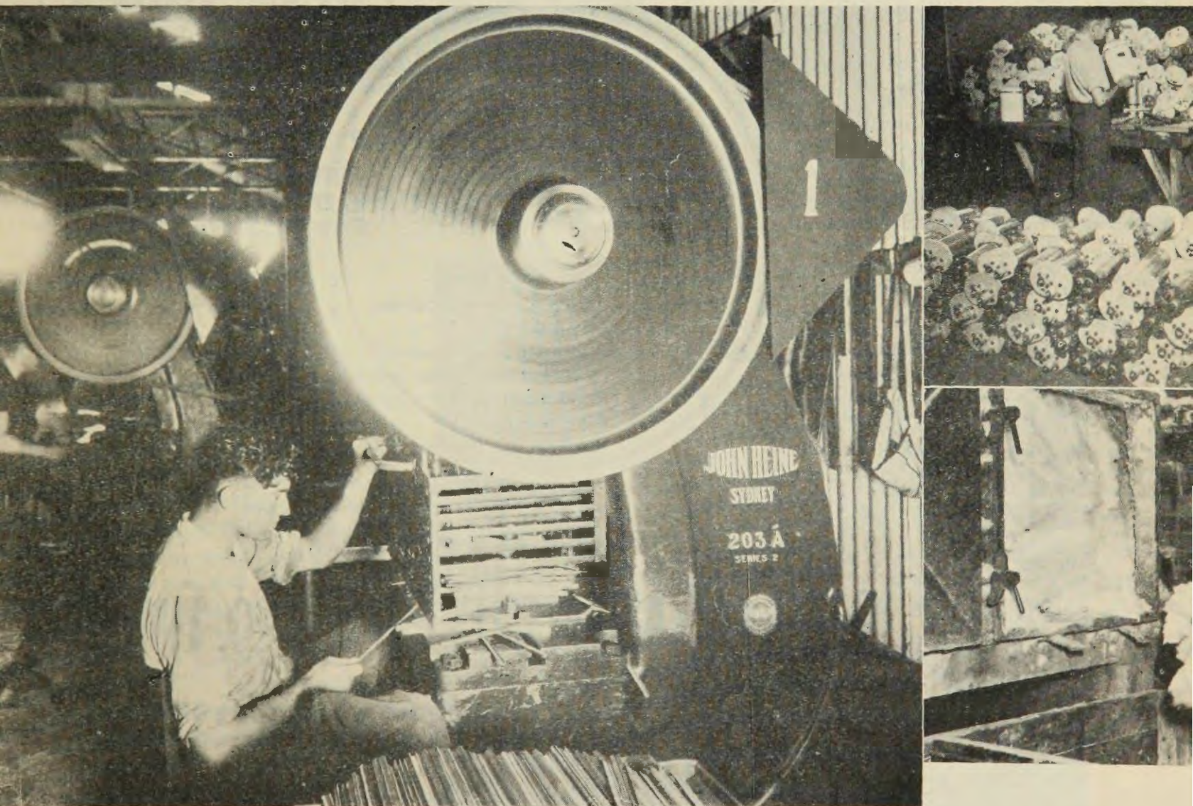
Interior views of the factory of J.C.W. Bridge & Co., at Mayfield
